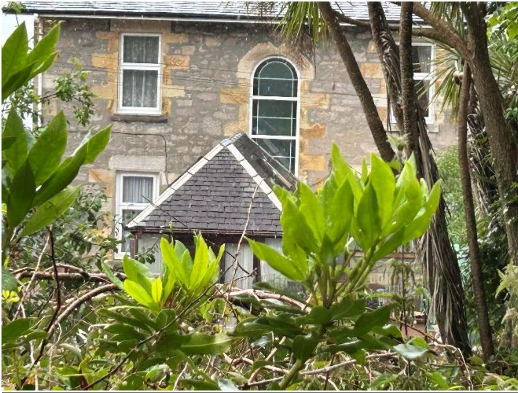
Rear elevation of 23 Crichton Road demonstrating uPVC replacement
