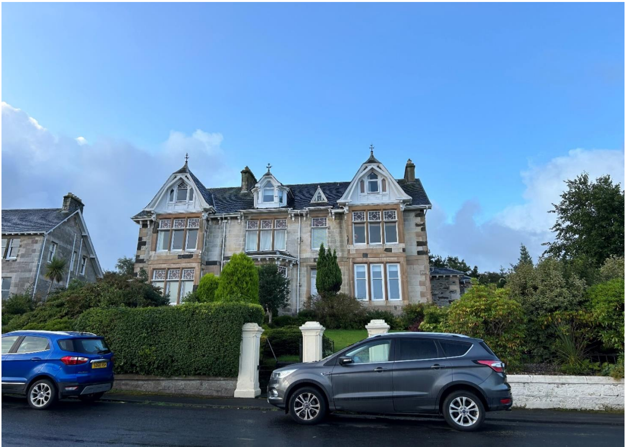
Front elevation of 19-21 Crichton Demonstration completely different fenestration and transom height in lower flat but approved REFERENCE NUMBER: 12/02280/PP
