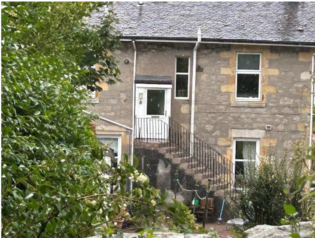
Rear elevation of 24 Crichton Road demonstrating uPVC replacement
