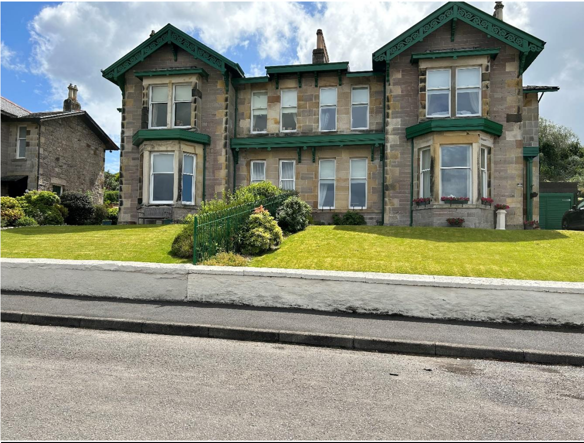
Front elevation of 28 -28 Crichton Road, demonstrates no difference in appearance of windows, lower flat 28, double swing, 27 Crichton Road sliding sash.
